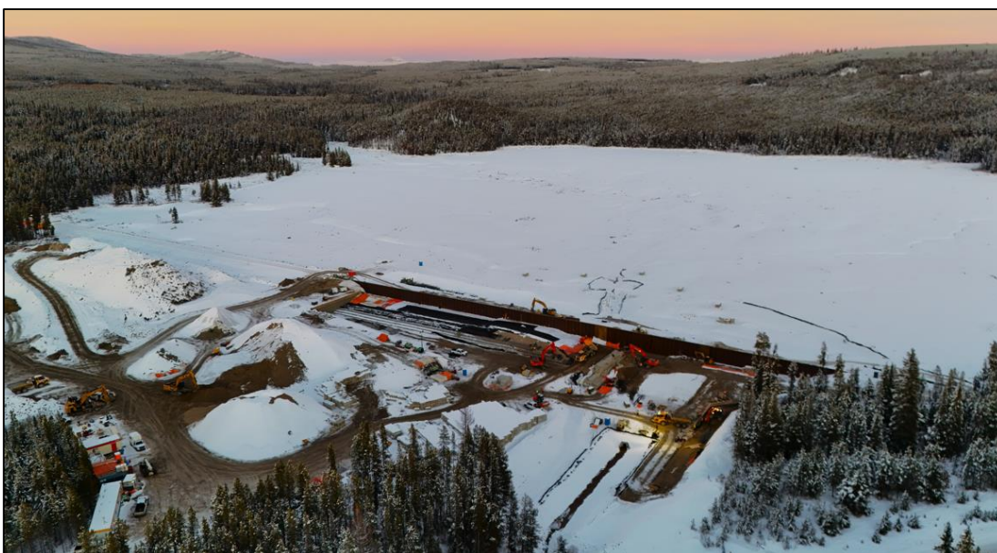
Figure 2: Site during Winter Construction
