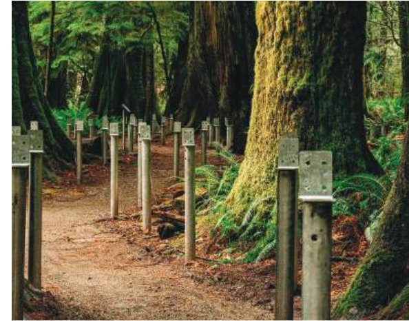
Low-Impact Footings (Pre-Boardwalk Installation)
