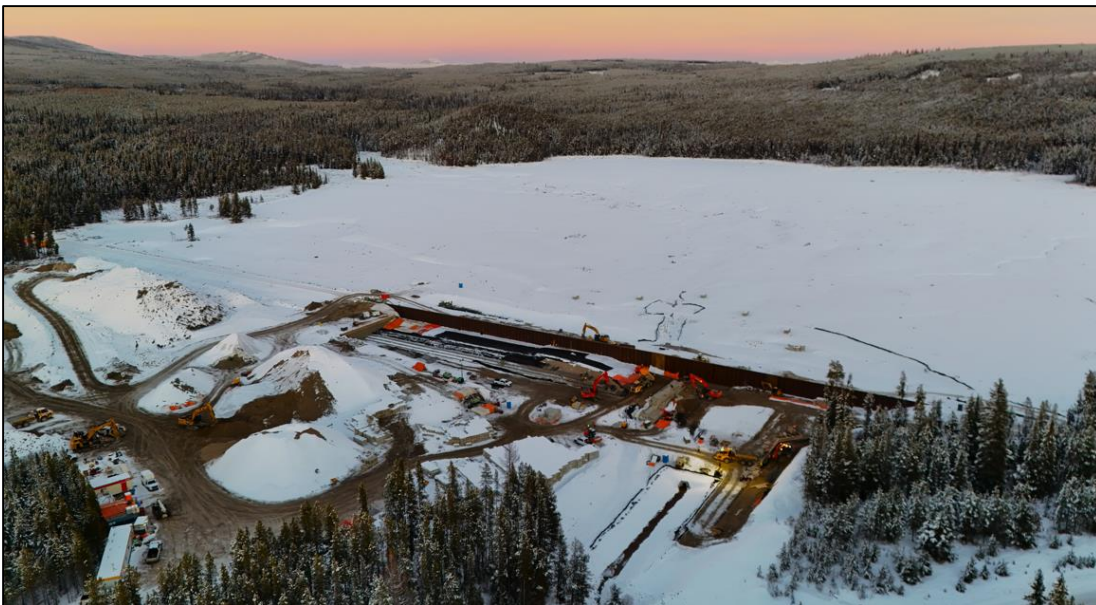
Figure 2: Site during Winter Construction
