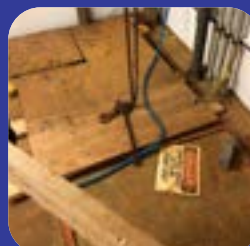
Wet well (sanitary sump) without proper hatch door
