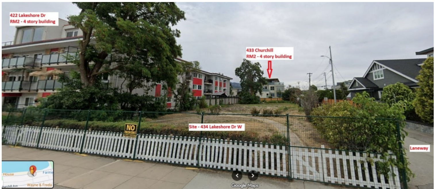
Figure 3 – Site and adjacent properties (courtesy of google maps)
